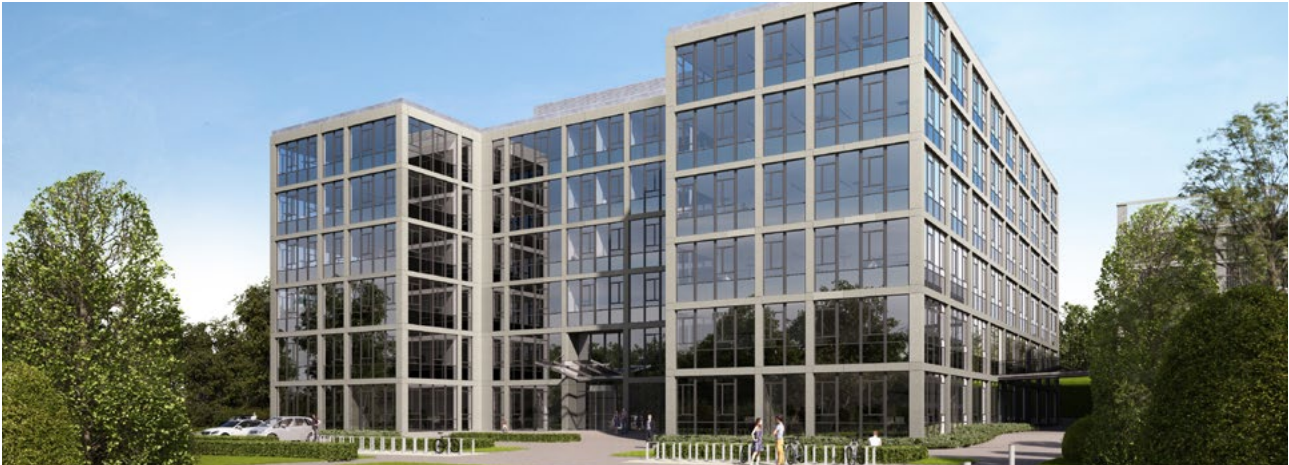
New SELLBYTEL building in the Tullnau Park, Nuremberg
